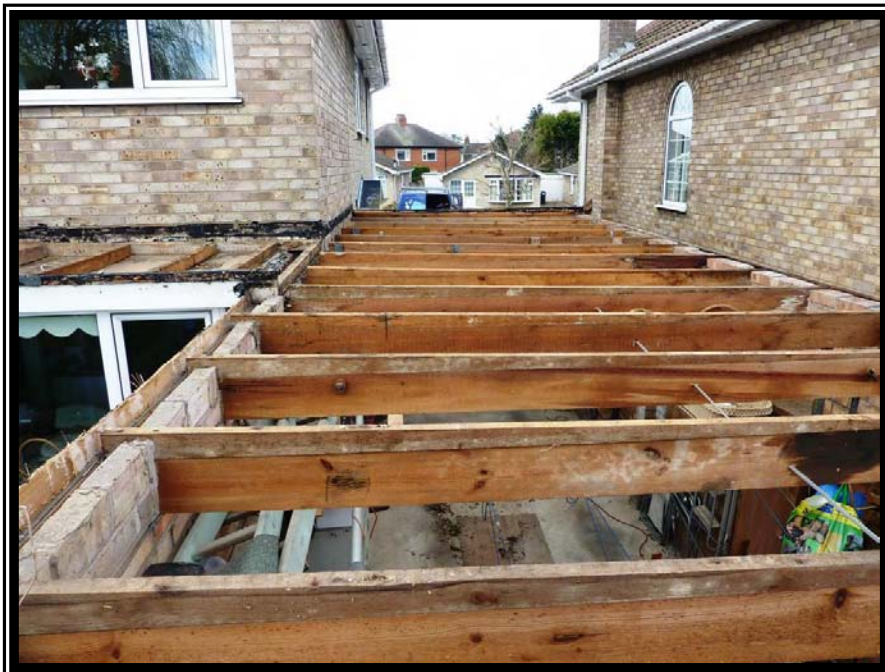
Roof stripped showing firings on top of joists
