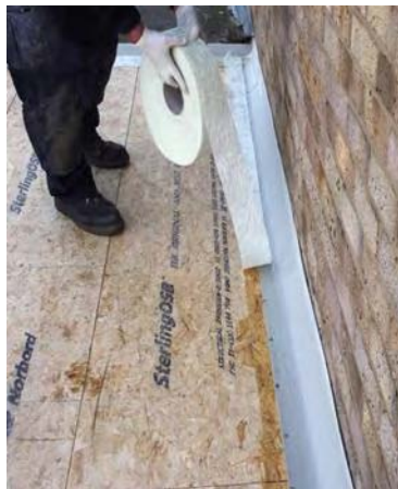
Bandage laid into resin
