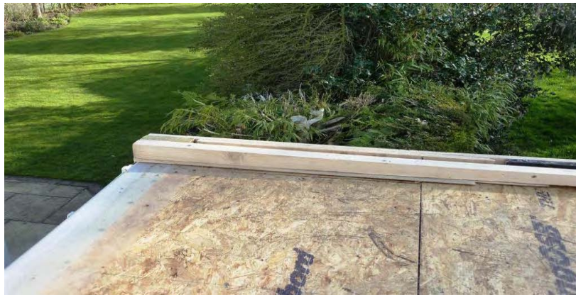
Reverse firring to level front and rear elevations
