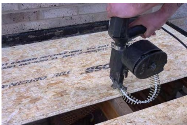
Decking fixed to support joists
