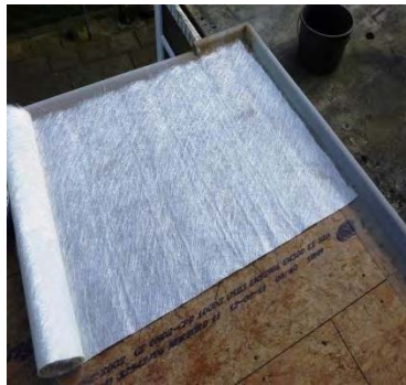
Mat laid into resin
