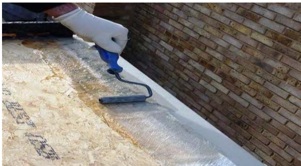
Use paddle to consolidate until transparent
