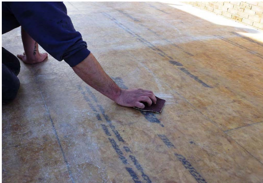
Lightly sanding cured laminate
