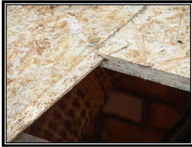
OSB3 tongued and grooved joint
