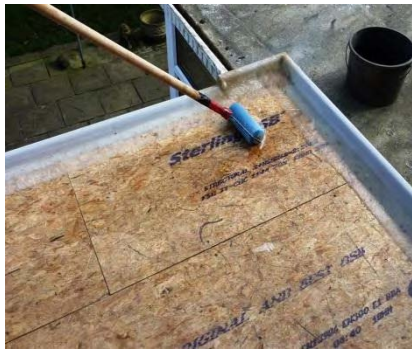
Base resin onto deck
